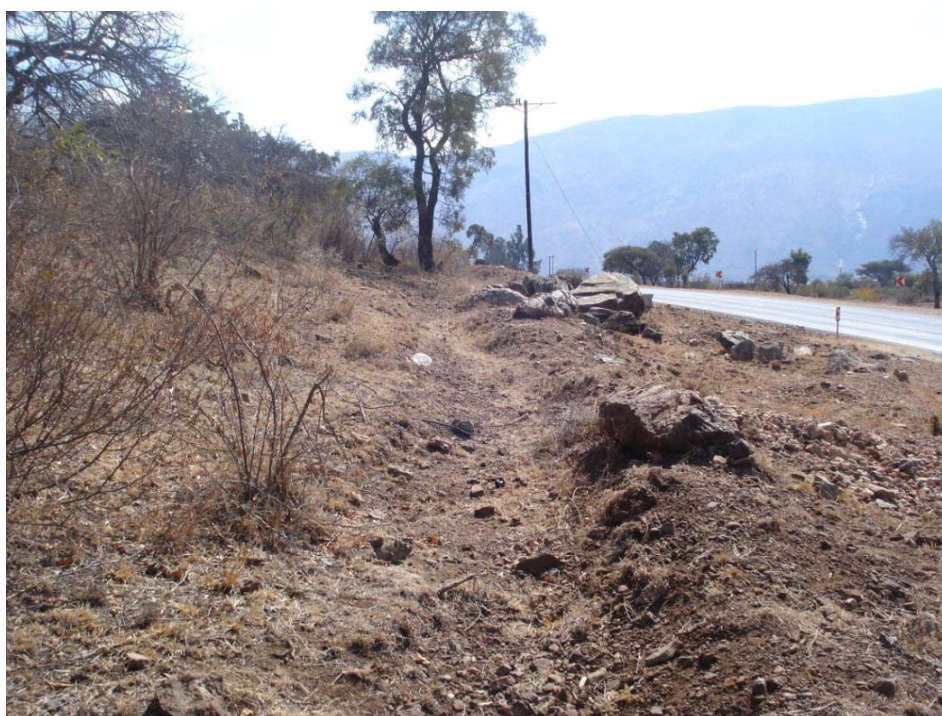
Photograph 10.7: Un-grassed side channels leads to erosion
