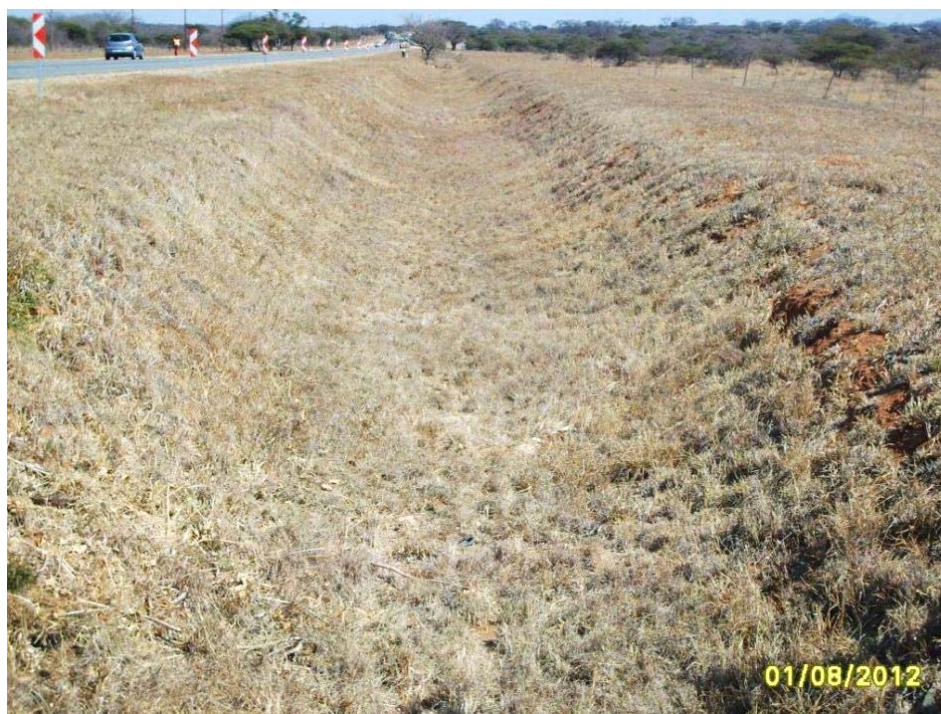
Photograph 10.4: Well-maintained lateral drainage channel
