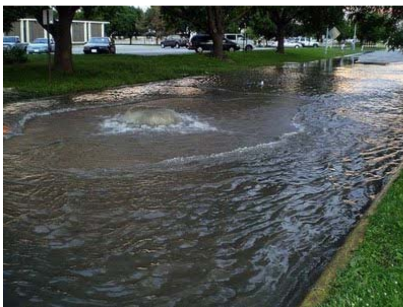
Photograph 9.4: Surcharging stormwater system
