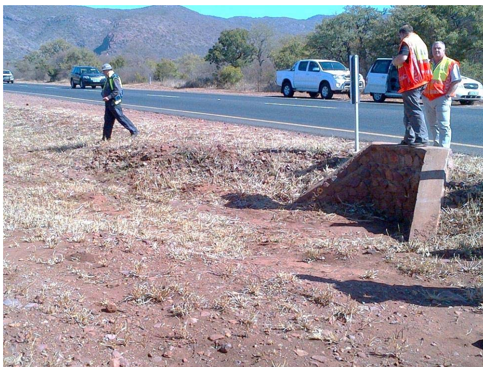
Photograph 10.1: An example of a culvert blocked by sedimentation on the N1 (Photo courtesy of Nuno Gomes)
