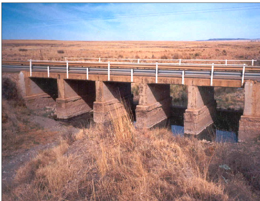
Photograph 8.4: Constriction scour (Courtesy of: Free State Department of Transport)
