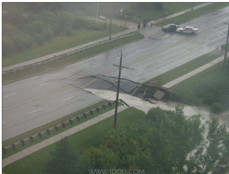
Photograph 12.3: Failure of a road surface due to “piping”, occurring around the culvert
