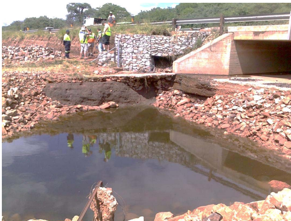
Photograph 10.3: Example of excessive erosion which occurred downstream from the culvert
