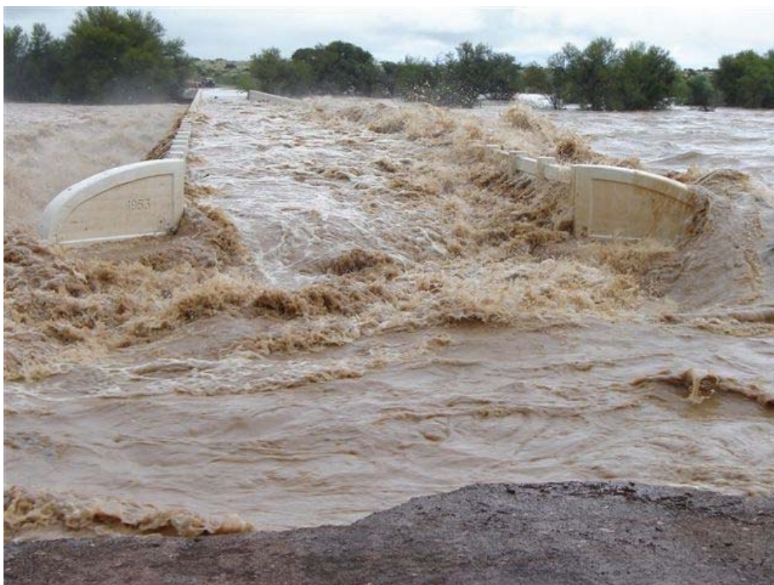
Photograph 11.1: Backwater curve due to damming at bridge
