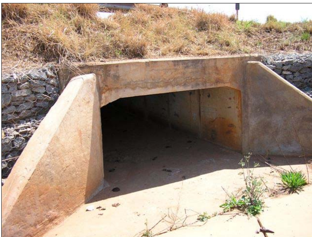
Photograph 7.2: Typical culvert with wing walls
