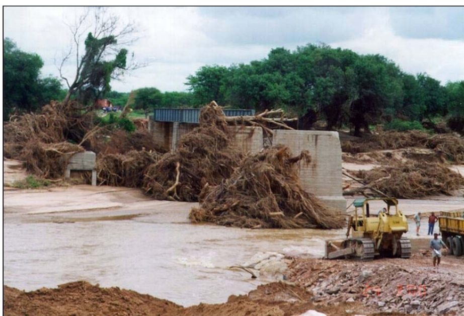
Photograph 8.1: Failure partly due to debris build-up
