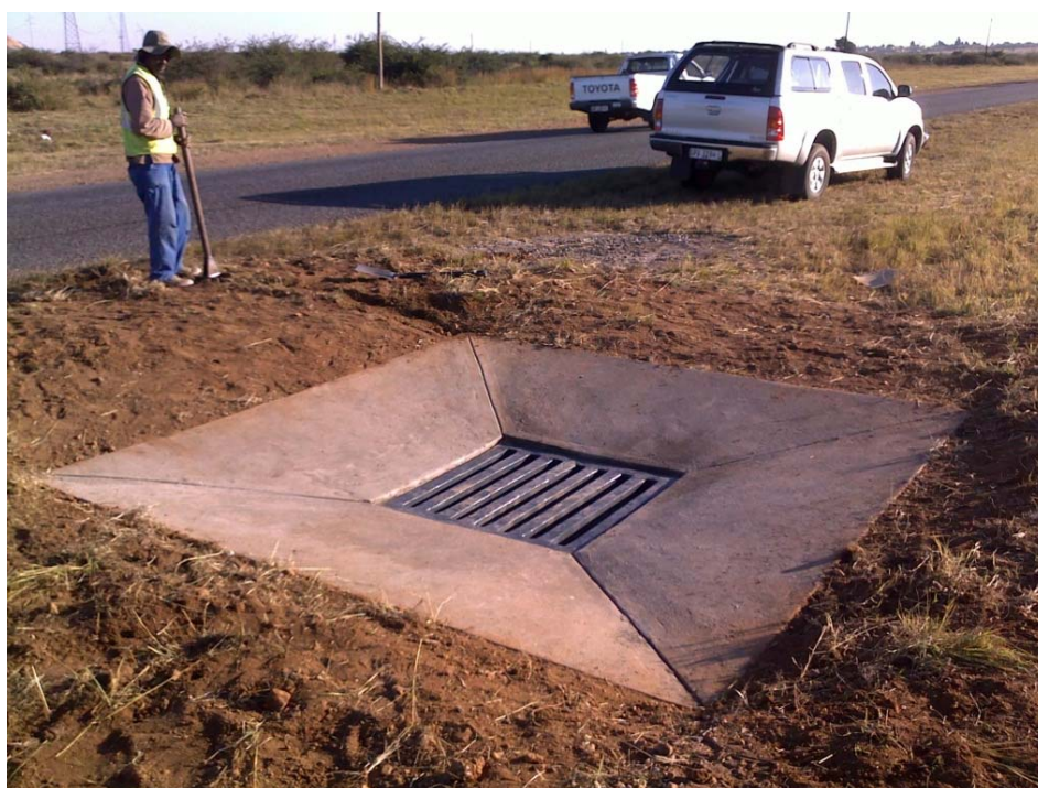
Photograph 10.6: Glass fibre drop inlet
