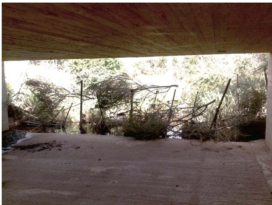
Photograph 10.13: Fences across the inlet of culverts will lead to undesirable blockages
