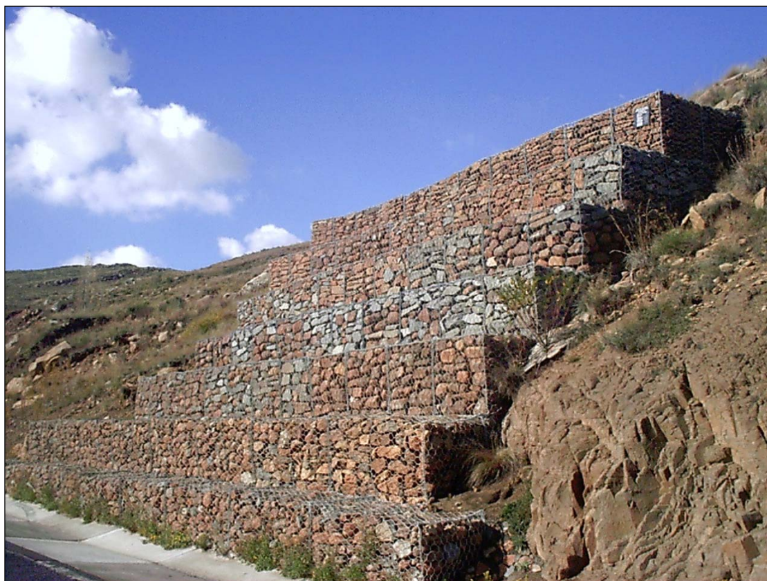
Photograph 5.7: Gabions used for bank stabilisation (Courtesy: Land Rehabilitation Systems)
