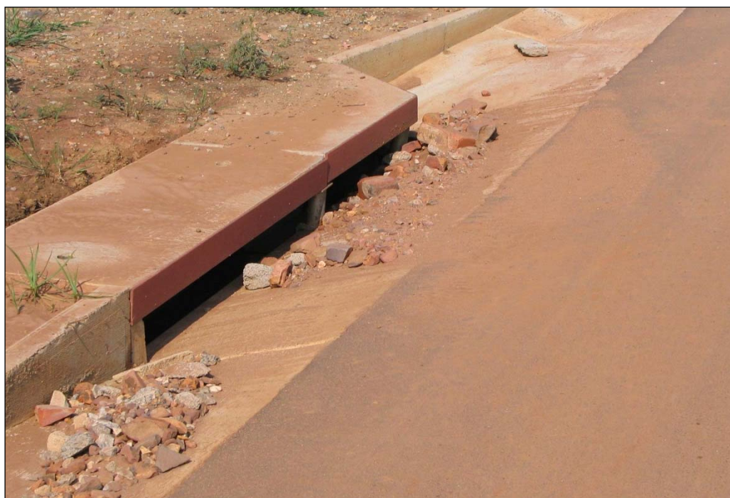
Photograph 5.2: Kerb outlet with deposited debris (Type III)
