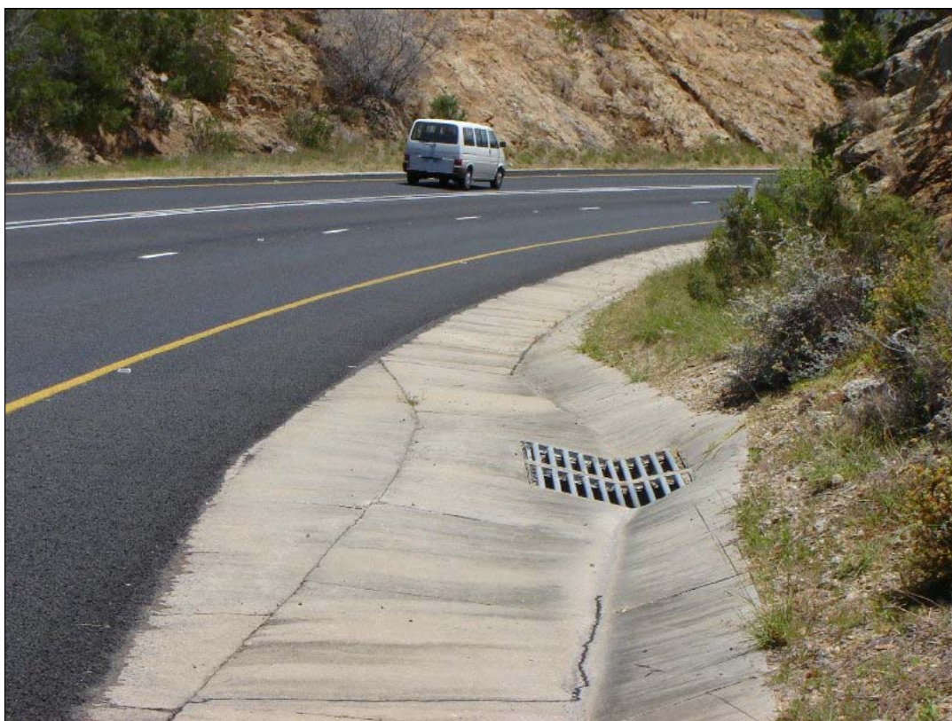
Photograph 5.3: Concrete side drain with grid inlet
