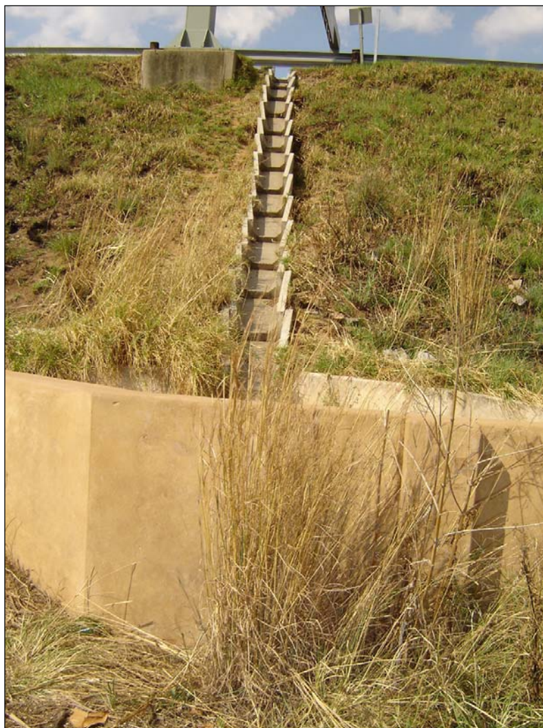
Photograph 5.11: Discharge chute, prefabricated blocks
