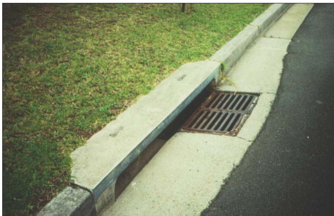
Photograph 5.4: View of a combined grid inlet and kerb inlet
