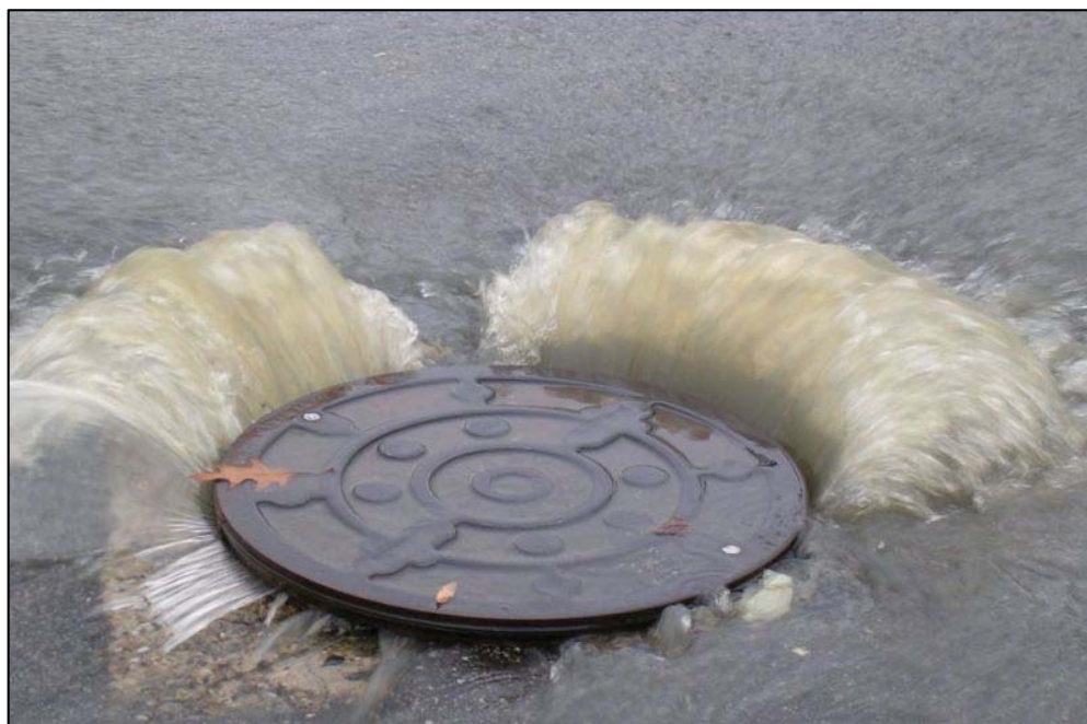
Photograph 9.2: Surcharging manhole
