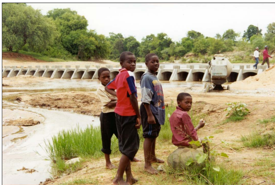
Photograph 6.1: A low-level river crossing provides safe access across the wide river
