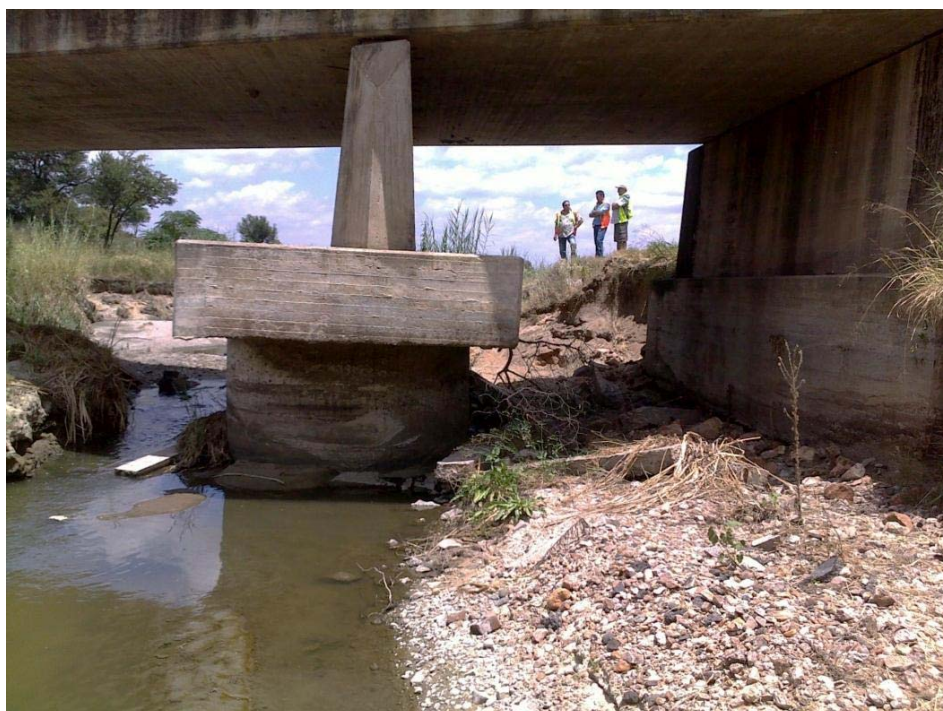
Photograph 10.9: Scour at a bridge pier
