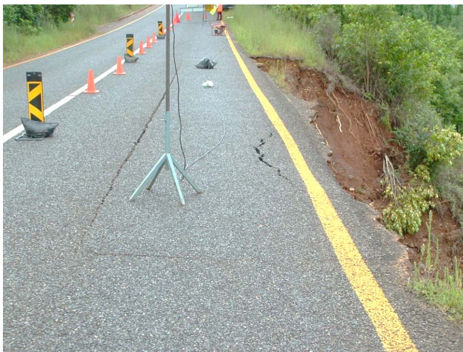
Photograph 10.12: Embankment failure
