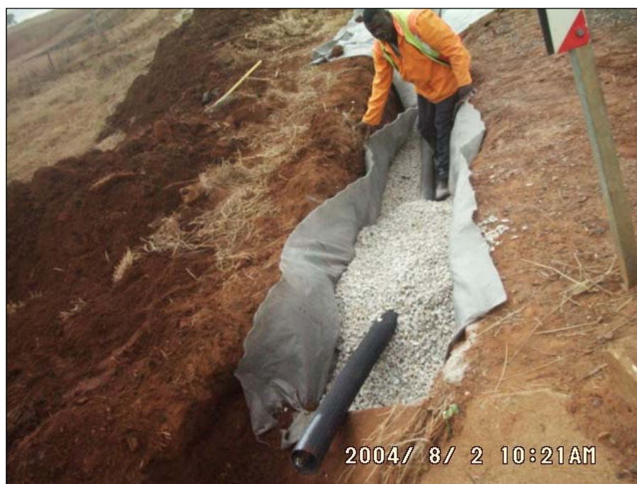
Photograph 12.2: Installation of sub-surface drainage to improve the drainage
