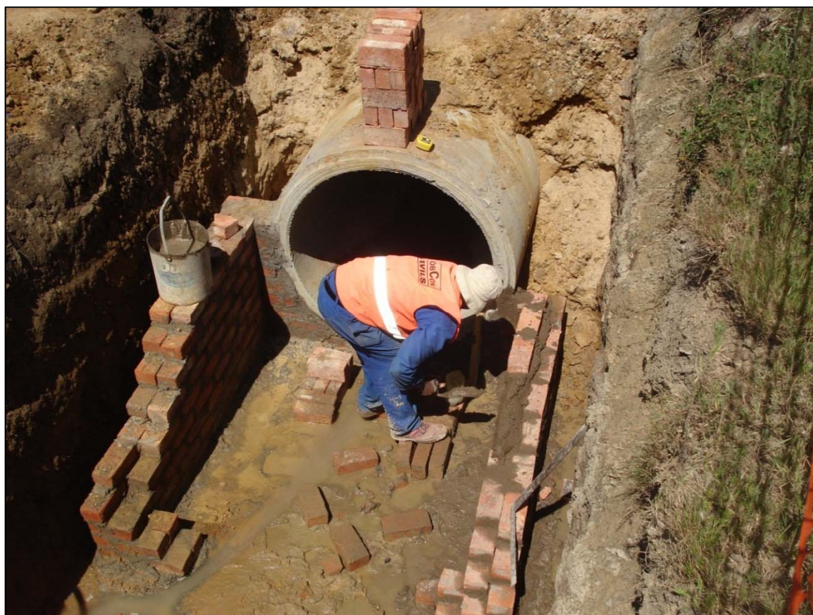
Photograph 9.3: Construction of stormwater access manhole (Courtesy of: MVD Consulting Engineers Southern Cape)
