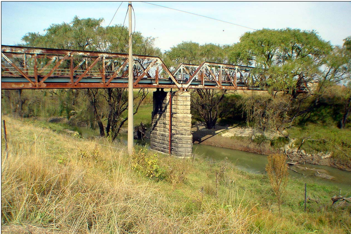
Photograph 4.2: River section in the Klip River. Estimated roughness = 0,10 m
