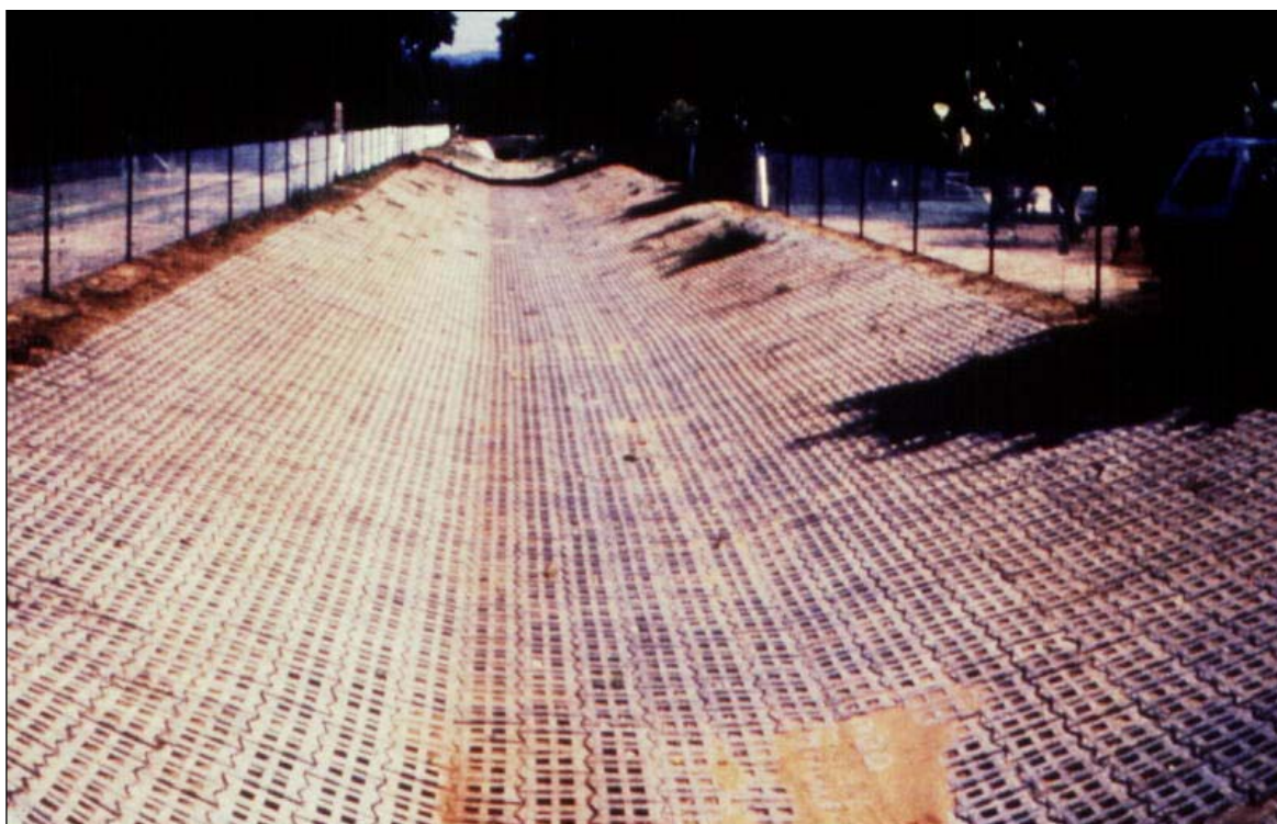
Photograph 5.5: Flexible concrete mattress for erosion protection in channels
