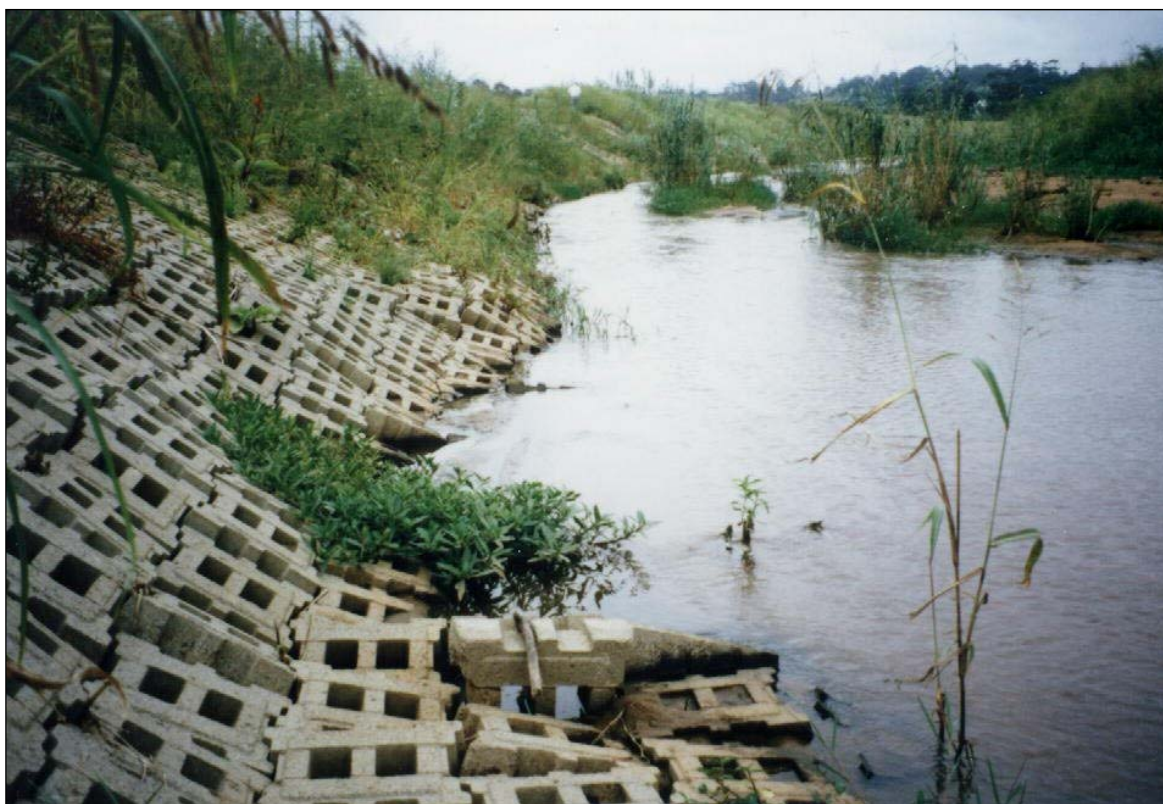
Photograph 5.6: Flexible concrete mattress failure due to weak supporting soils
