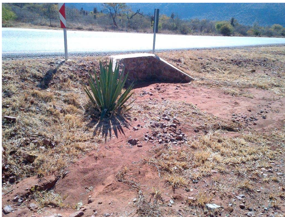
Photograph 10.8: Siltation of culvert inlets
