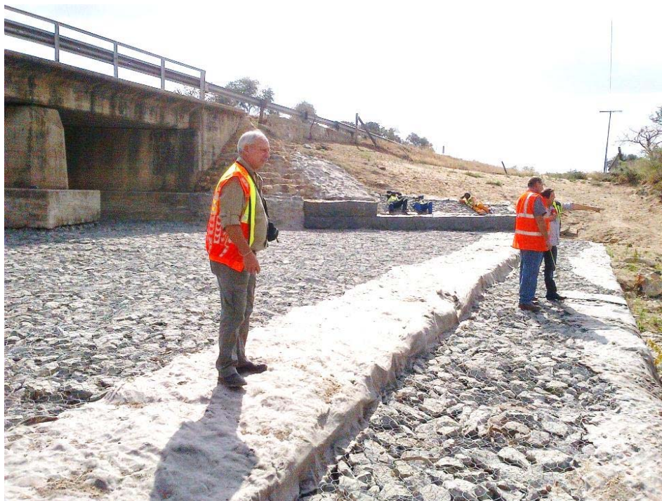
Photograph 10.10: Repair of scour damage which occurred at bridge shown in Photograph 10.9
