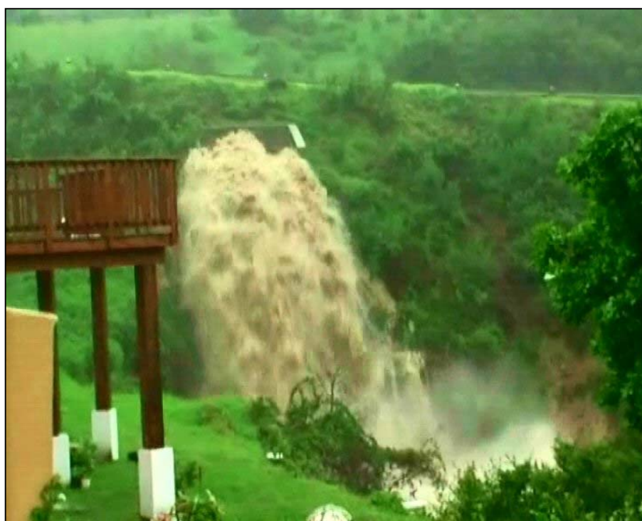
Photograph 9.1: Pressurized flow in conduits (Courtesy of: MVD Consulting Engineers Southern Cape)
