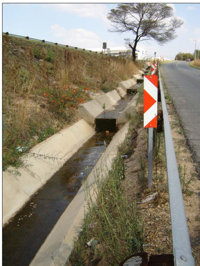
Photograph 5.10: Stepped energy dissipator along the N3
