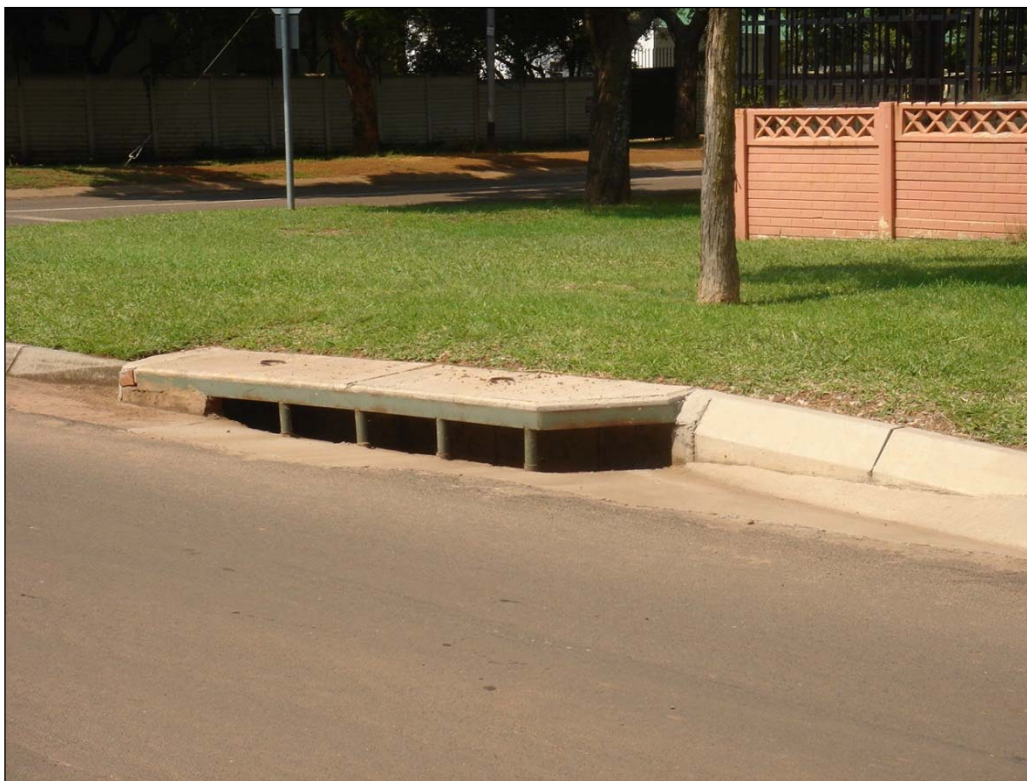
Photograph 5.1: Detail of a typical kerb outlet with a transition section (Type III)
