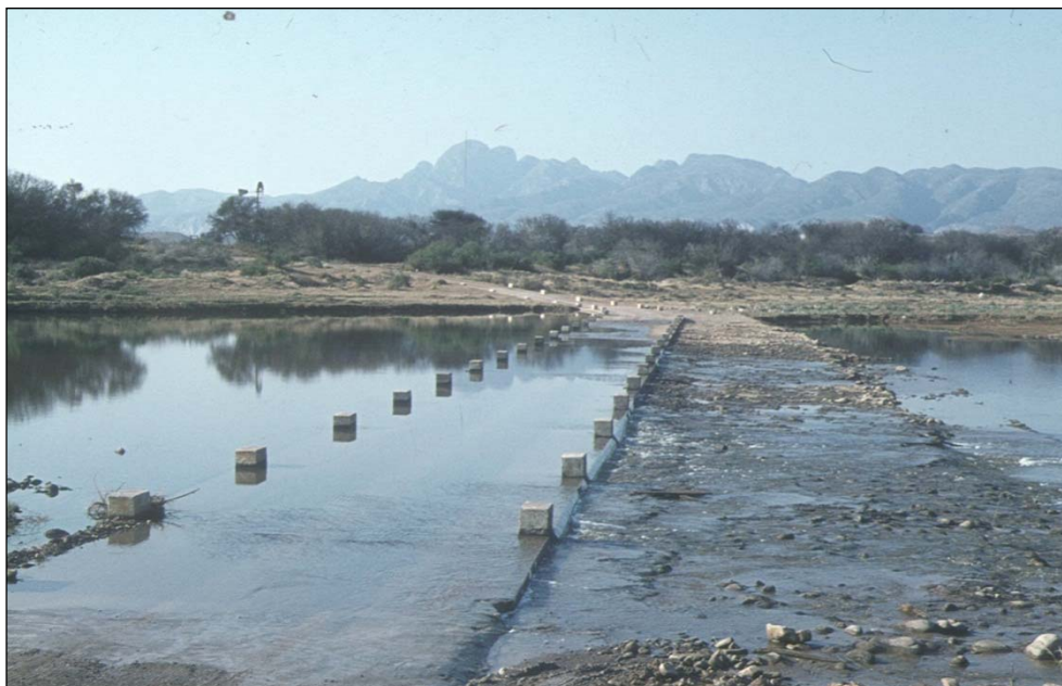
Photograph 6.3: A low-level crossing near Steytlerville, showing the guide blocks
