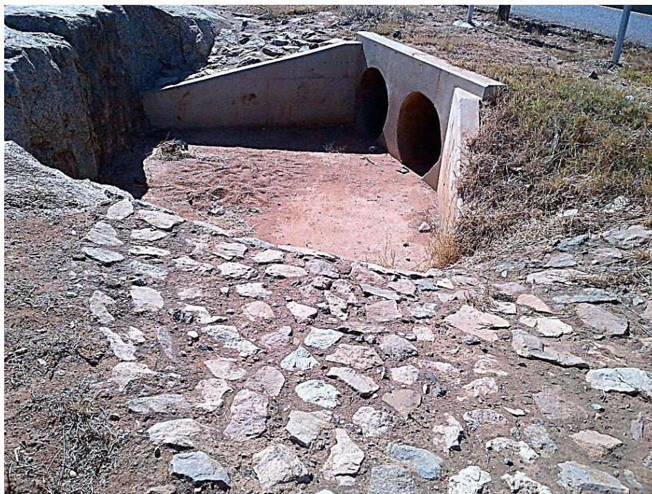
Photograph 10.2: Alteration to the culvert inlet to prevent siltation (Photo courtesy of Nuno Gomes)
