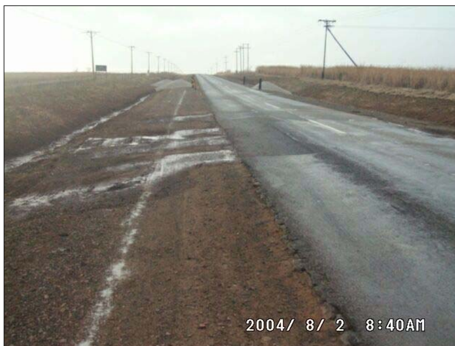
Photograph 12.1: Typical conditions associated with poor sub-surface drainage design
