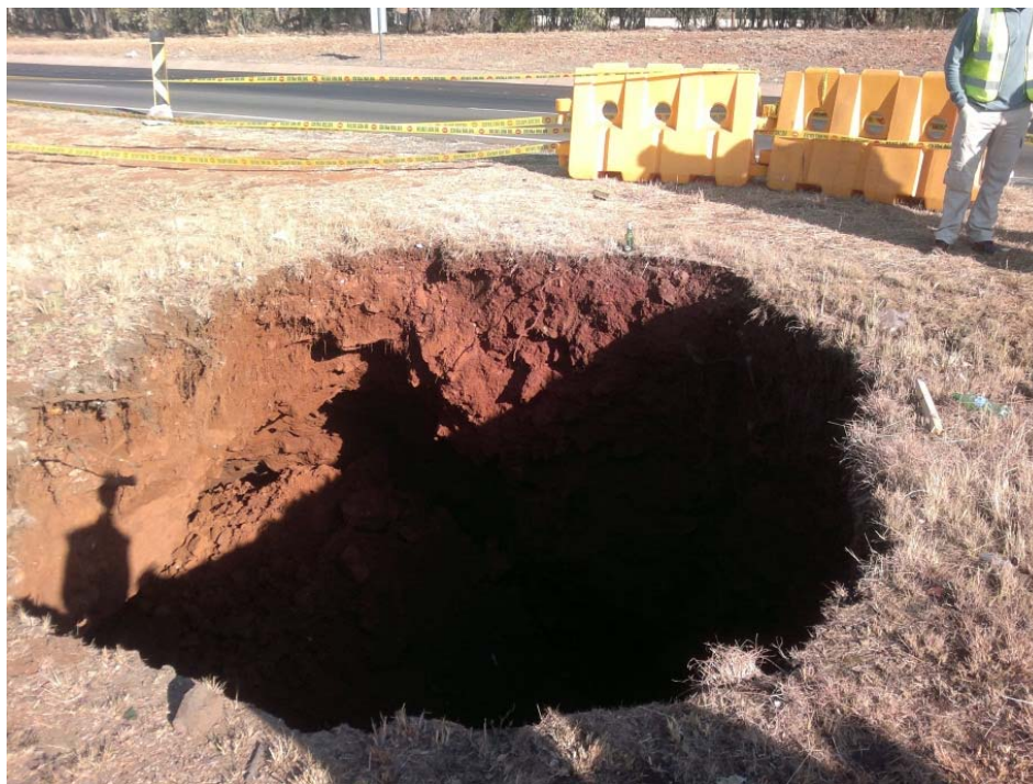
Photograph 10.14: Sinkhole formed on the median of the N14
